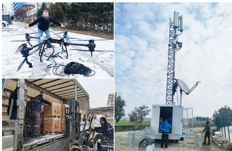
Huawei engineers work side by side with carriers to rapidly get networks back online in the affected areas in Türkiye.
